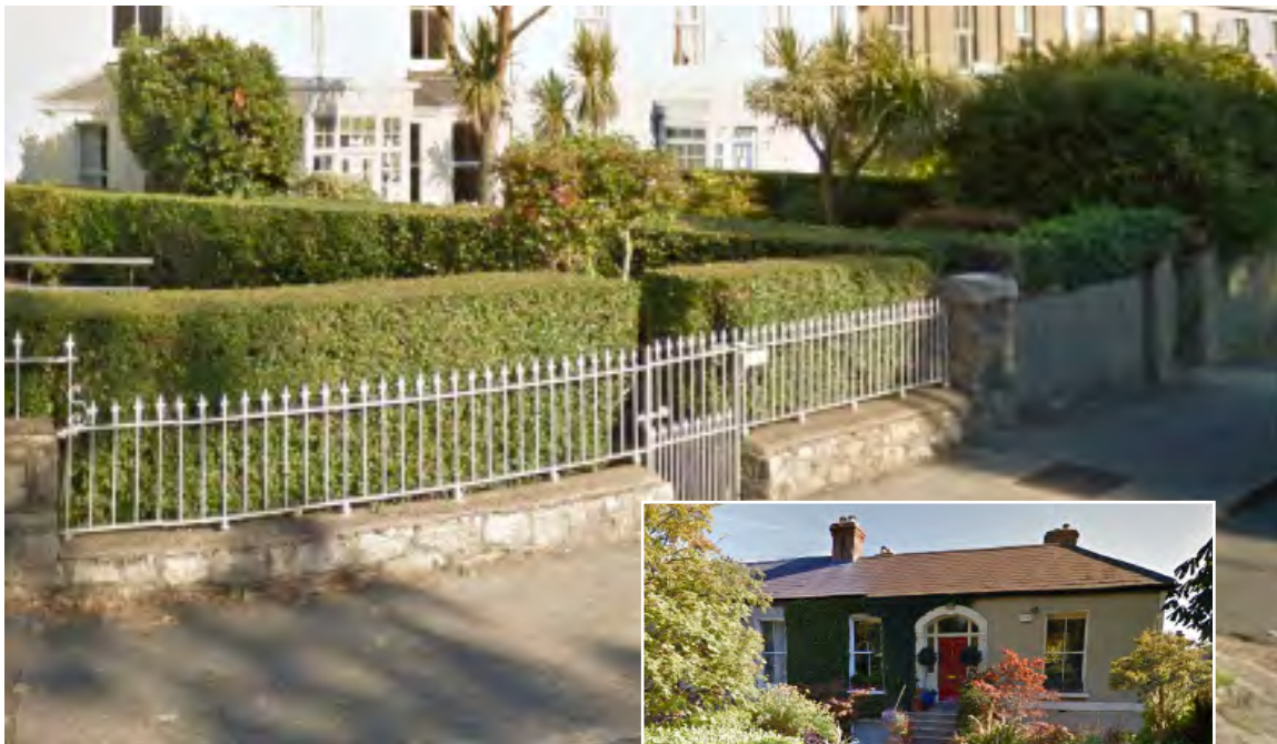
Gardens and railings intact - Novara Terrace Inset: Preserved features - Sidmonton Square - Google Earth
