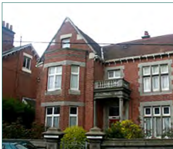
Wellington House, Novara Avenue - Building Survey of Ireland.
