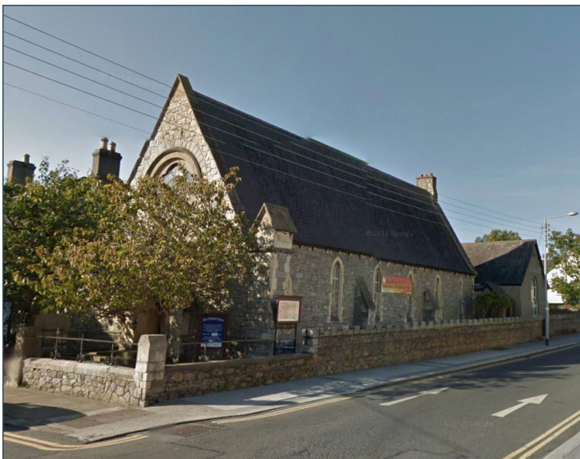
This Methodist Church, on the corner of Florence Road and Eglinton Road, was built in 1864 from granite rubble with sandstone dressings. According to NIAH it is “well preserved and combined with the group value of the adjoining manse it adds much to both the streetscape and the historic character of the area”.
